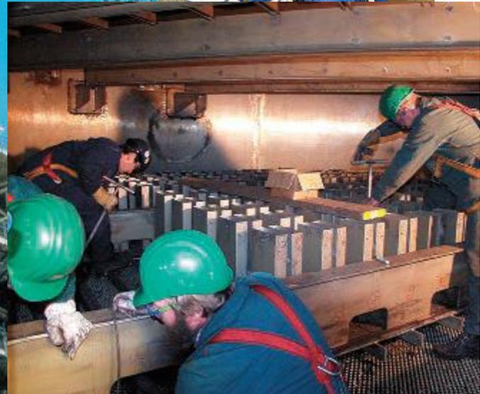
*Installation of the liquid distributor*
