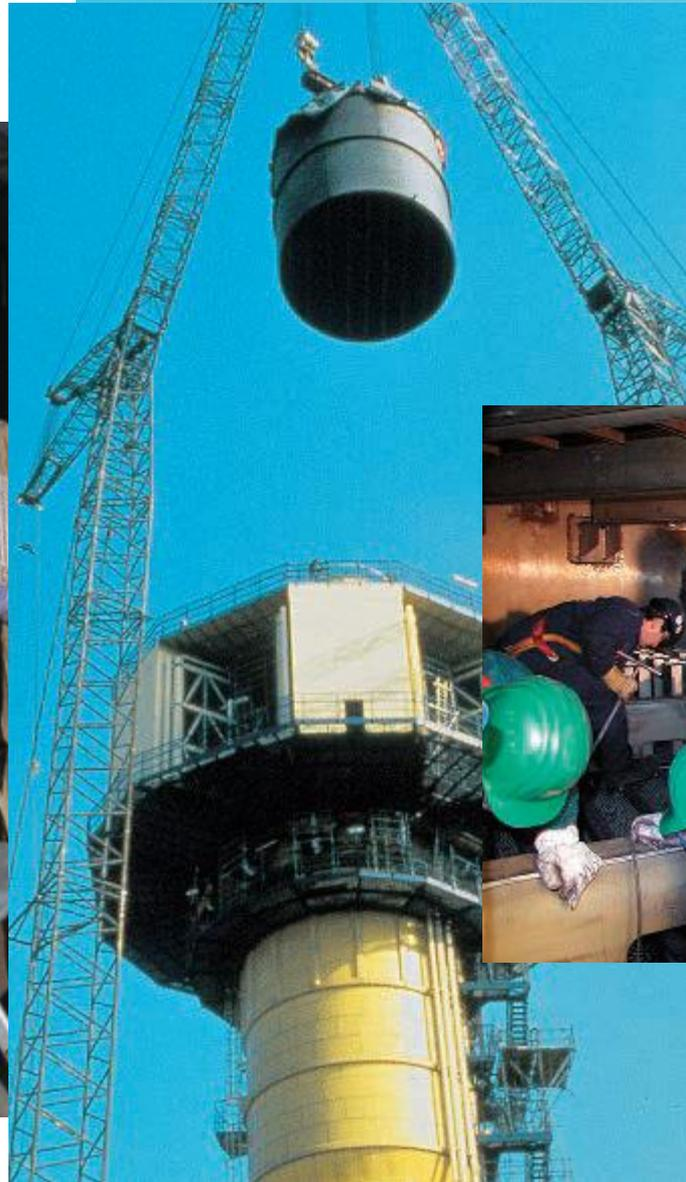
*The column sleeve is lowered into the column with two cranes. Weight: 100 tons*
